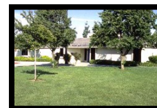
Valley High School 6300 Ehrhardt Avenue
