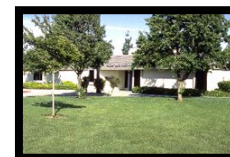
Valley High School 6300 Ehrhardt Avenue
