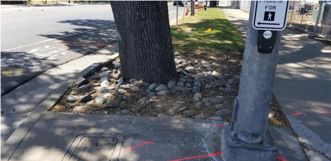
May 2021. Notice there is no cobble embedded in the concrete, as shown in the photo on the bottom of the previous page.
