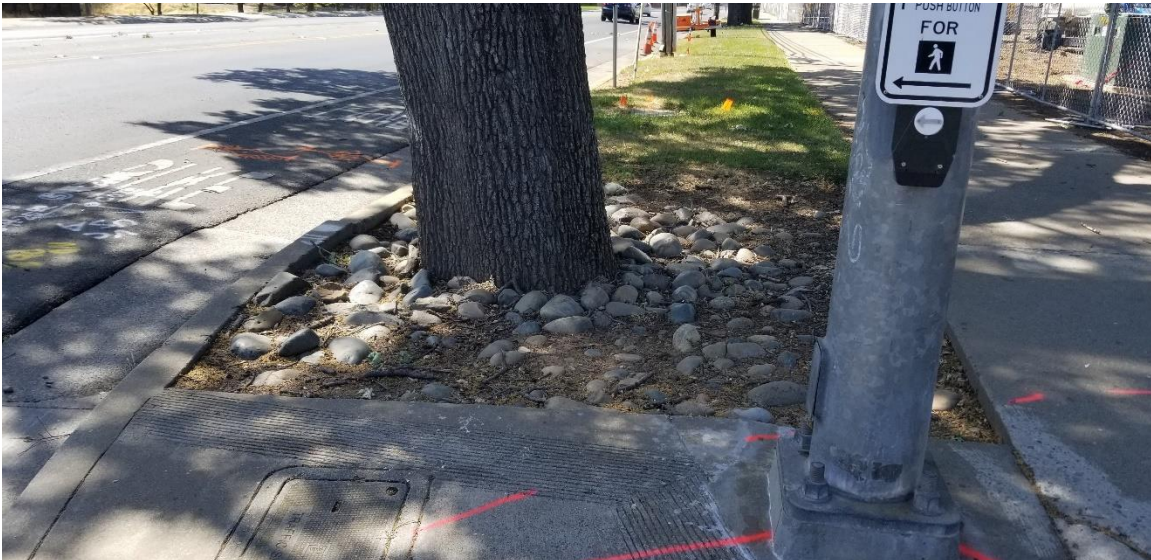
Tree #152 above has an absence of root flare, and the root collar appears buried by the cobblestone. In addition, the USA (Underground Service Agency) markings beneath the dripline suggest the utility trenches may need to be accessed, which would result in root damage to the subject tree. An ISA certified arborist should be present to observe the excavation beneath the dripline and evaluate the extent of the damage.
